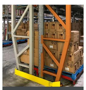
The DAMO PRO CAN can be used to repair damage to the front and back columns of a rack.
